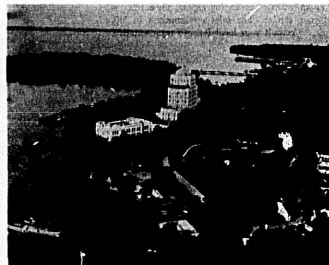
VIEW OF THE FLAMINGO HOTEL, MIAMI BEACH, FLORIDA
